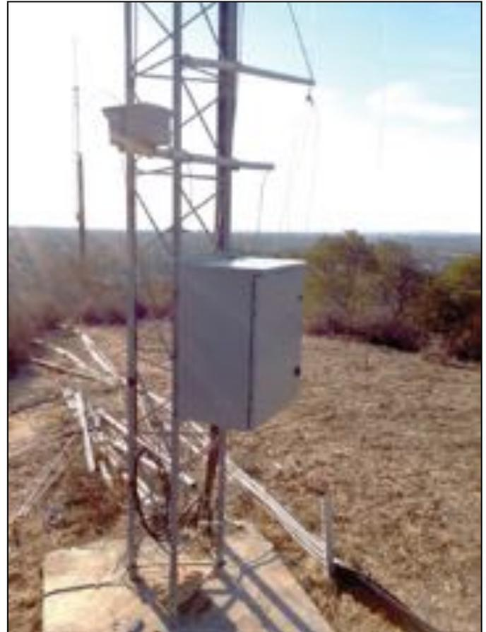
**Figure 2: Mesa HF junction box installed on the Rohn tower**
