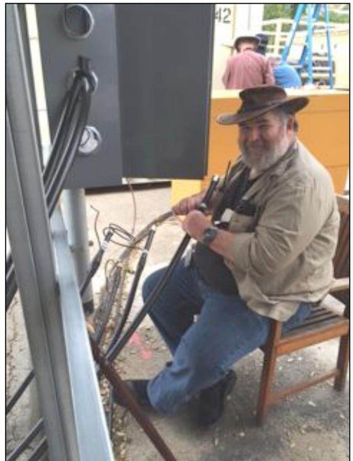
**Figure 9: Chris Carson KE6ABQ installing grounding kits on the new hard lines going up to the Mesa.**
